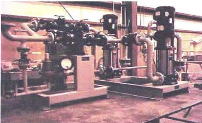
HEI Dual Pump & Filter Station Assembly with back-up capabilities
