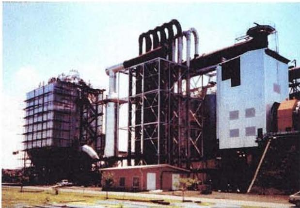
SONIQUENCH System using Ultimix spray nozzle technology upstream of a baghouse at a metals plant.
